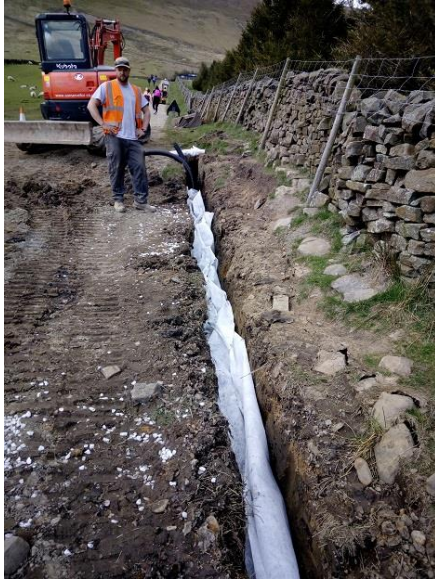
Adding new drains to the lower path, and the erosion of the zig zag section prior to work starting April 2021
